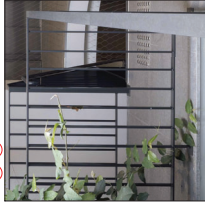
MS.1 NEW VERTICAL SLAT - NEW PAINT COLOUR TO MATCH WALL BELOW / ADJACENT
